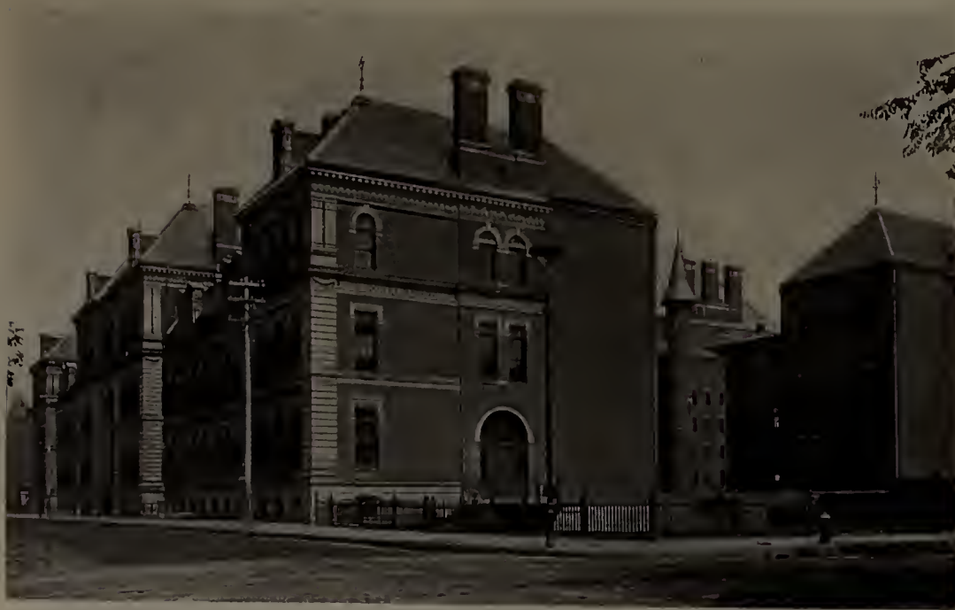
BOYS' LATIN AND ENGLISH HIGH SCHOOL, Warren Avenue. These buildings cost $750,000. George A. Clough was the architect.
